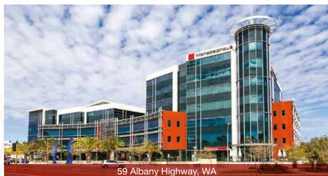
59 Albany Highway, WA
