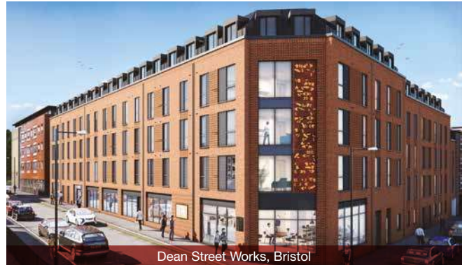
Dean Street Works, Bristol
